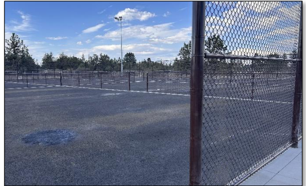
New courts under development, July 13, 2026.
