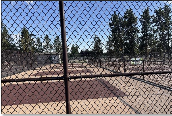
Court repairs in progress, July 13, 2026.
